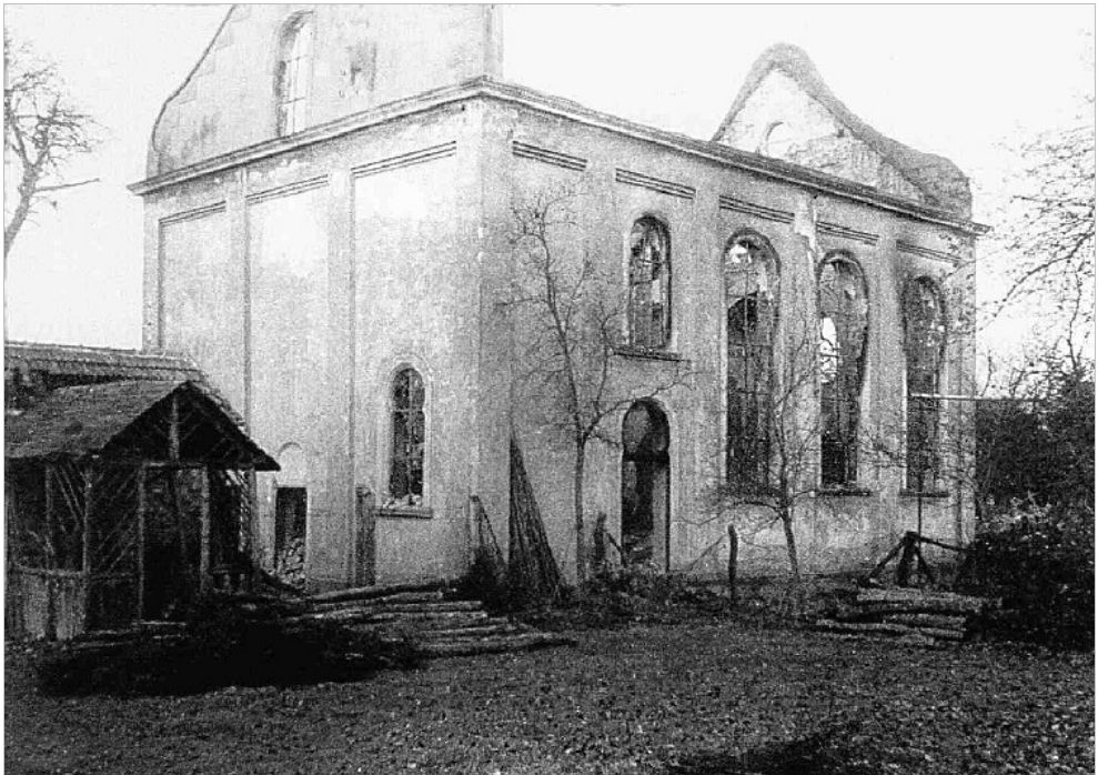
The venerable House of the Lord of Burghaun's Jews after the November crime of Nov. 10, 1938. The ruin was razed and the sandstones were used to built a small railroad station for the Huenfeld-Treischfeld railway. The destruction of their religious center was at the same time the end of Burghaun's Jewish community/ congregation.
